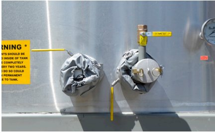
Dual Heated/Insulated Outlet Valves
